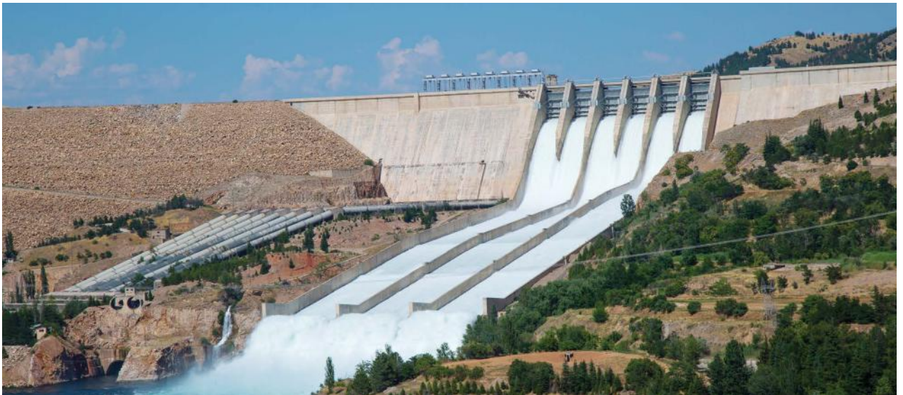
Keban Dam, Elazig
