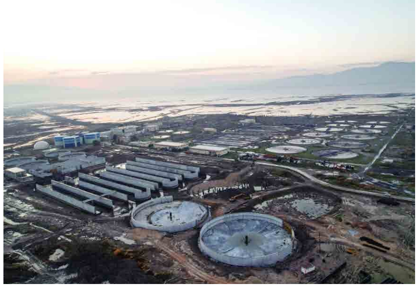
Cigli Wastewater Treatment Plant
